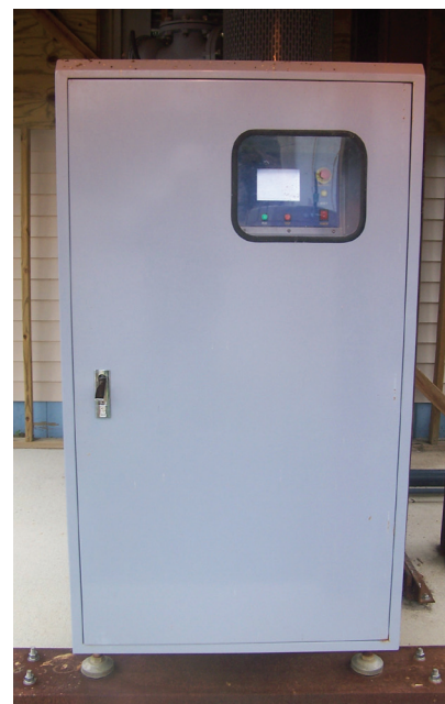
The James River Wastewater Treatment Plant (Newport News, Va.) uses a turbo blower adapted from jet engine technology.
