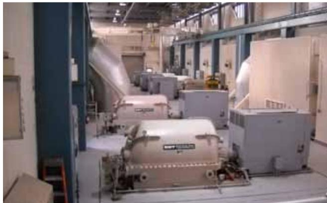
**The Mill Creek Wastewater Treatment Plant is scheduled to have its six multistage centrifugal blowers replaced with single-stage, integrally geared centrifugal blowers with dual vanes for inlet and outlet air control. This project is scheduled to be finished in 2015. MSDGC**
