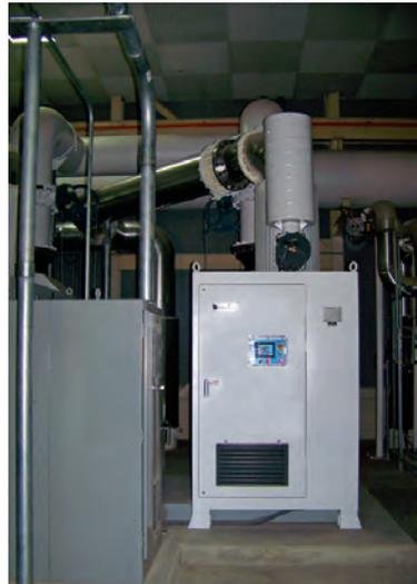
Two 300 hp APG-Neuros turbo blowers will save the Scottsdale Water Campus wastewater treatment plant about 47.5 million kWh over the next 10 years, a reduction of about 40 percent. The units can be adjusted to match wastewater flows. The \$771,000 cost was covered by a U.S. DOE grant through the American Recovery and Reinvestment Act.
